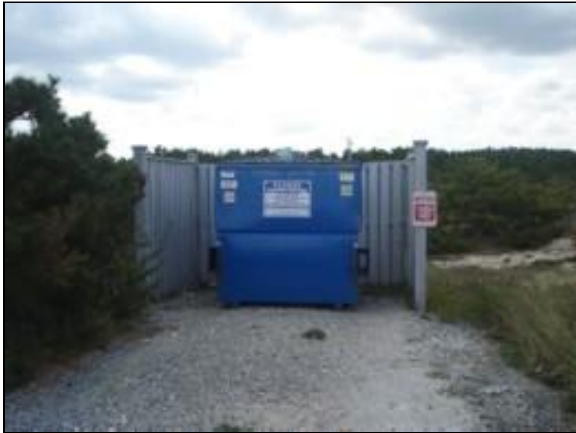
Photo #1. Dumpster Enclosure
