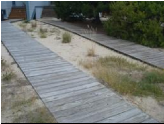
Photo #3 Walkways to Units – Not in Study
