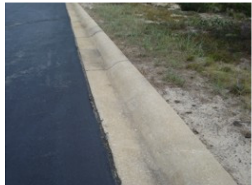
Concrete Gutter
